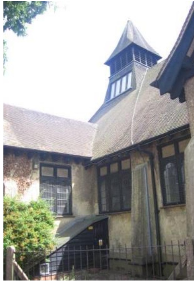
St Nicholas Church, Battenburg Avenue
